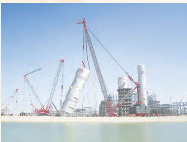
Fig. 6 The ALE SK190 lifting a 2200 Tons Pressure vessel in Ruweis, UAE.
