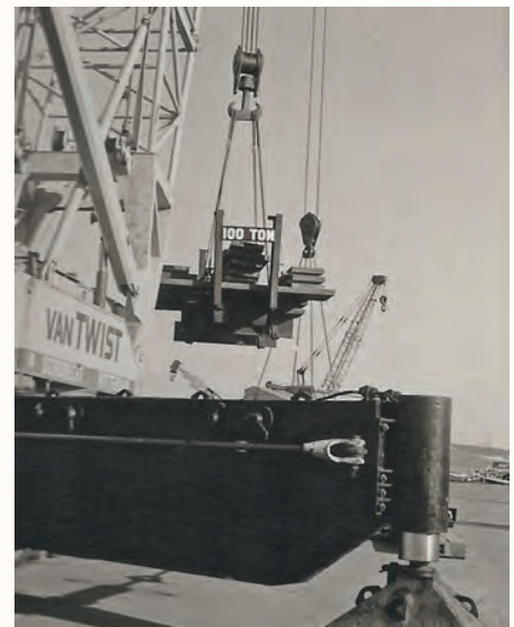
Fig.2 The Gottwald MK500 from 1968 lifting a 100 tons test load
