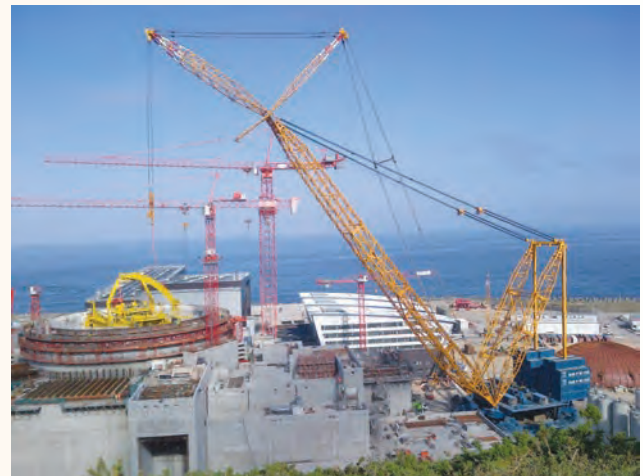
Fig.9 The SGC-120 lifting the dome of the Flamanville EPR reactor building, which weighs 260t and has a diameter of 43m.
