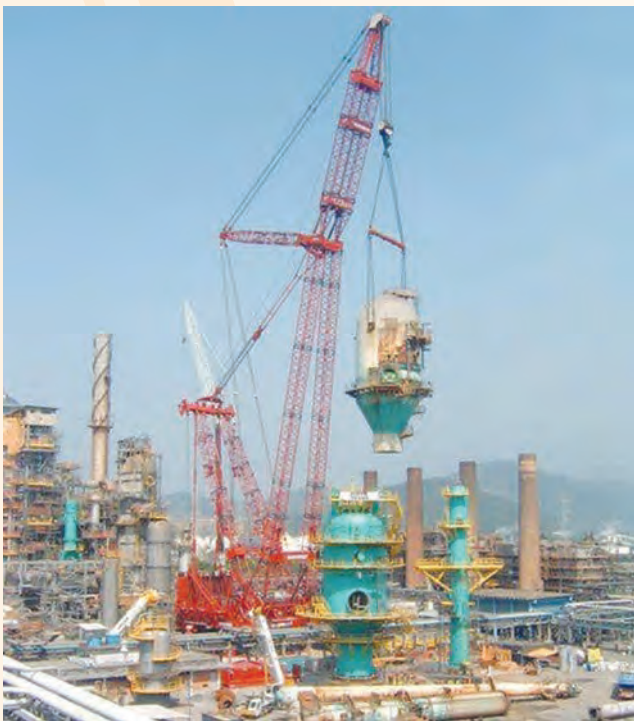
Fig.3 The Mammoet PTC200-DS lifting a Pressure vessel
