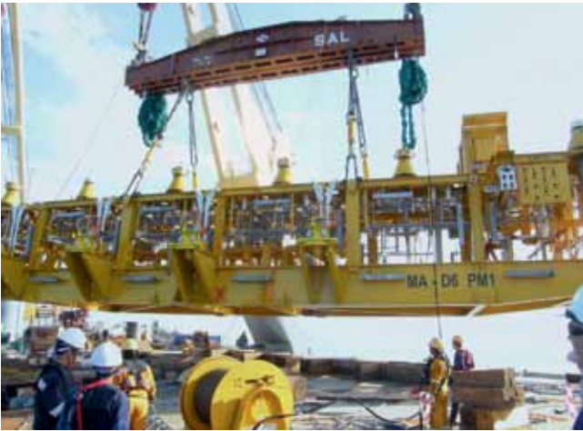
Manifold Overboarding – MA D6 Project
