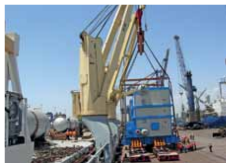
Lifting arrangement Boiler Block
