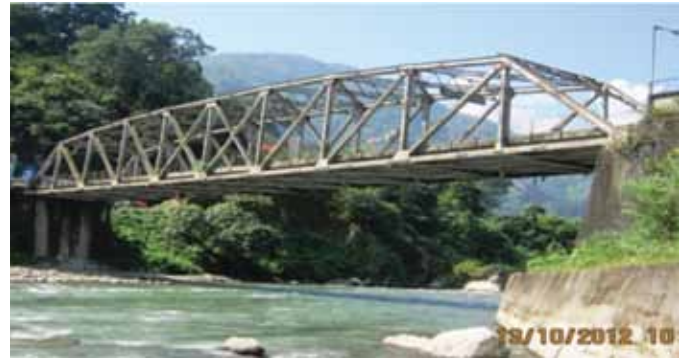
Fig 1: Rangpu Steel Truss Bridge (Taken From upstream side)
