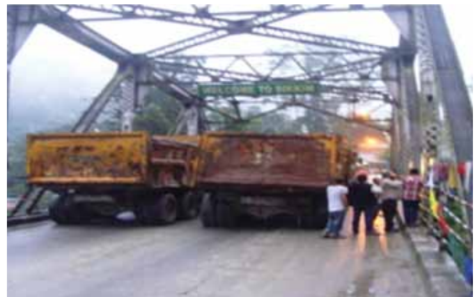
Fig 15: Stage-IV Loading of Load Test on Rehabilitated Rangpu Bridge (Taken From Seveok, West Bengal side)
