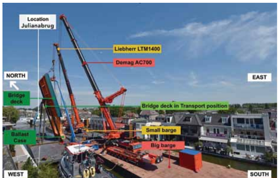
FIG.5 The Liebherr LTM1400 and Demag AC700 just before the incident
