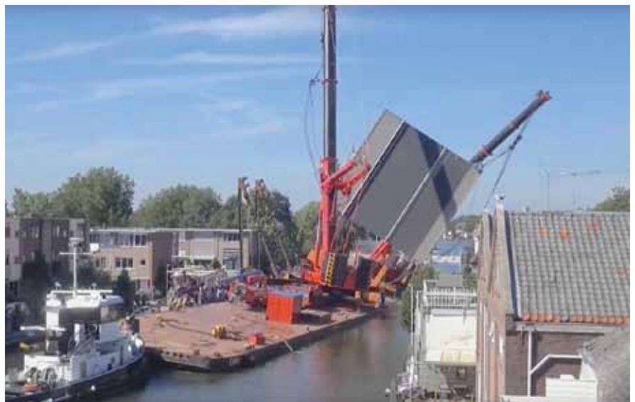
FIG.3 Due to insufficient Stability of the barge, the list increased and main boom of the Liebherr collapsed
