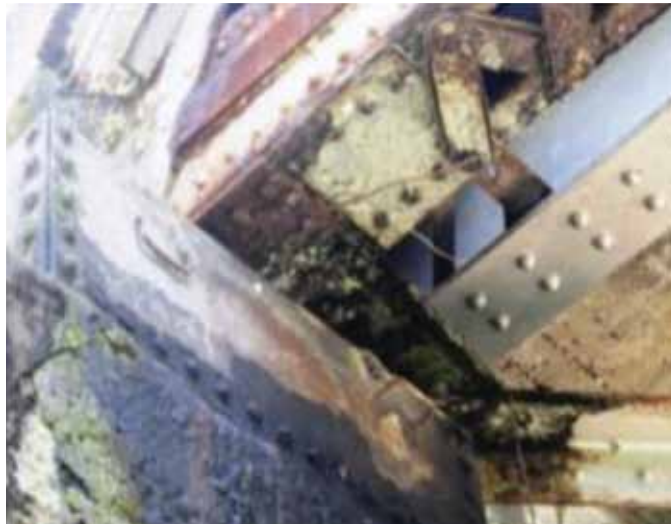
Fig 3: Immense rusting/corrosion of bottom chord at bearing location
