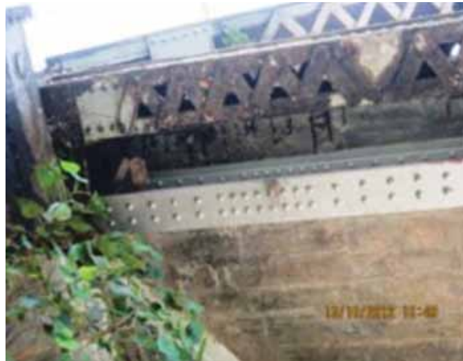
Fig 4: Rusting of exposed deck slab r/f. & rusting/scaling of bottom chord members
