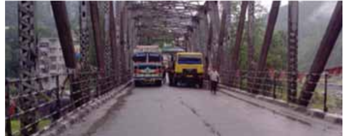
Fig 7: Carrying out of Load Test on Rangpu Bridge (Taken From Sevoke, West Bengal side)
