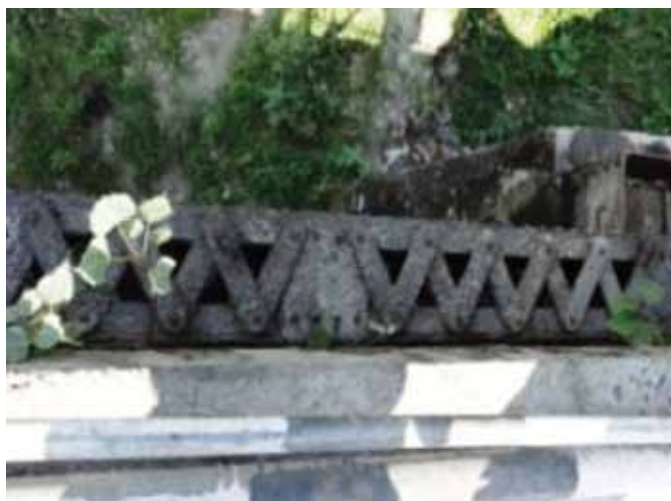
Fig 5: Corrosion of bottom chord truss members.
