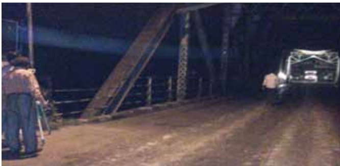
Fig 12: Stage-I Loading of Load Test on Rehabilitated Rangpu Bridge (Taken From Rangpo, Sikkim side)
