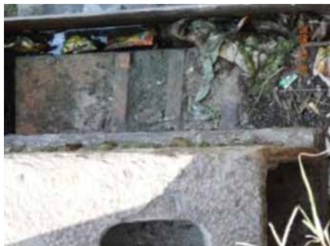
Fig 6: Metallic bearing filled up with non/biodegradable waste and water.
