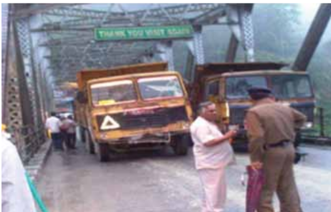
Fig 14: Stage-III Loading of Load Test on Rehabilitated Rangpu Bridge (Taken From Rangpo, Sikkim side)
