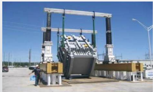
Figure 40. shows the upending of a transformer in progress.
