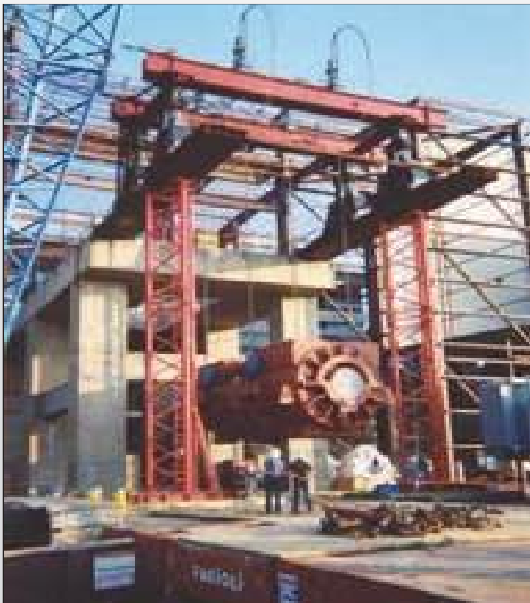
Figure 42. Hydraulic gantry used for the tailing operation of a vessel.
